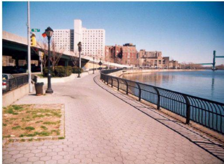
Figure 14 - Site of the 96th Street Power Station on the East River in New York. Photo by R. Lobenstein, 2007.
