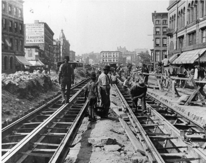
Figure 1 -The mechanical San Francisco type cable was introduced on Broadway Avenue in 1892, giving New Yorkers improvements in travel and comforts over horse-cars. Courtesy of A. Lonto.
