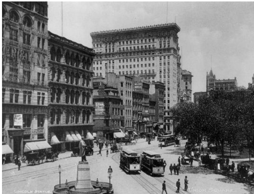
Figure 12 – Streetcars traveling on Broadway at Union Square in 1904 were propelled by electricity from the slot in the road. Courtesy of A.Lonto.
